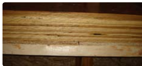
Glue lams are laminated support beams consisting of many thin pieces of wood glued together. You cannot drill or notch these beams.
