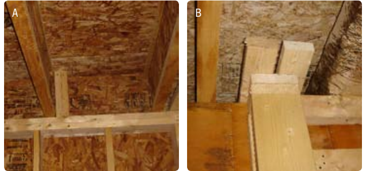
(A) Load-bearing walls intersect directly with the floor above. You'll see the wall run continuously up to the ceiling. (B) Non-bearing walls don't intersect directly with the floor above. In this image, there's enough room for a heating duct to run between the wall and the ceiling.
